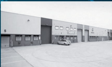
F. WALTHERR ELECTRICS LTD, UNITED KINGDOM
