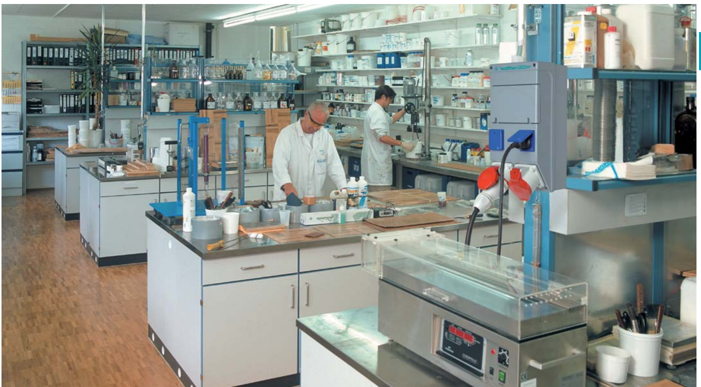
Figure: Use of a chemically-resistant socket combination in the laboratory
